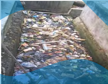
Garbage in Main drains
